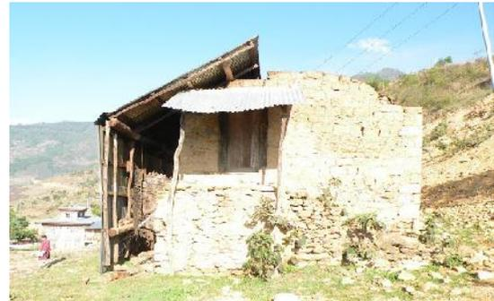
Fig.4 Wind damaged roofs(2011)
