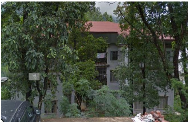
Figure 1: View of the Building
